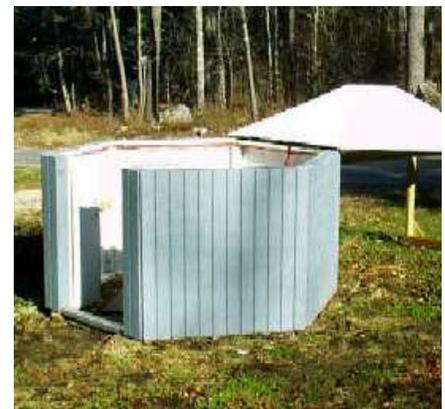
The structure is made primarily of 3 sheets of T1-11 siding; three 3 sheets of 3/8-inch plywood for the roof; 10 fir 2x4s; 8 PT 2x4s; 6 (3/16xX2 inch) aluminum flat stock (bent to 25°); and one-half sheet of 3/4-inch plywood.
